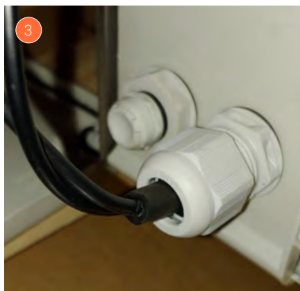
Blind plug to mount the LED cable.
